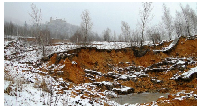
Fig. 7: January 2011 landslides on the edge of open-pit coal mine in the immediate vicinity of the Krušné Hory fault scarp, with the Jezeří castle on the horizon.
