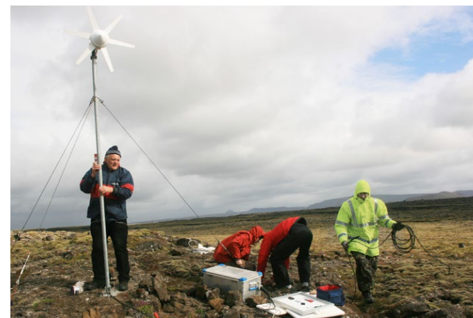
Fig. 6: Installation of seismic station STH of the network REYKJANET on the Reykjanes Peninsula (southwest Iceland) in September 2013. The REYKJANET stations are equipped with broadband sensors Güralp a Gaia data acquisition systems, and supplied by combination of solar panels wind generators.
