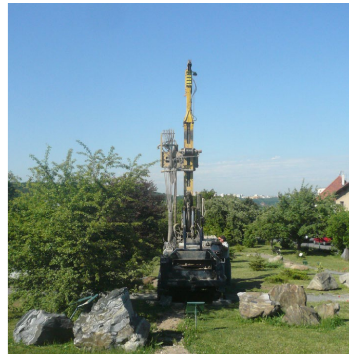
Fig. 10: Drilling the borehole for the new geothermal observational site – Spořilov 3, in the Geopark of the Institute of Geophysics, May 2011.
